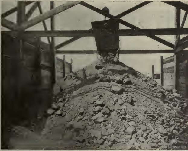
BUCKET DUMPING A LOAD OF MINE-RUN COAL AFTER CARRYING IT OVER 120 FEET FROM CAR
